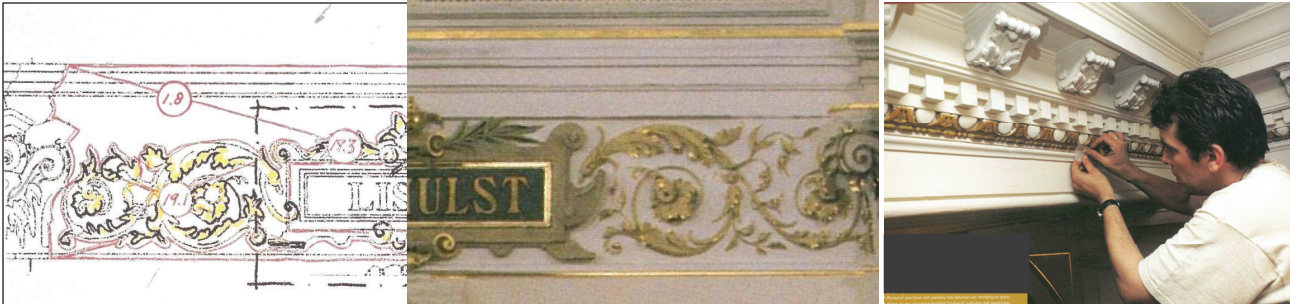
Figure 6. Gold plating of the ornamentation (9)
