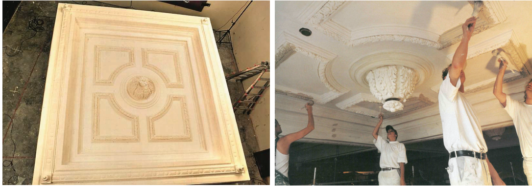
Figure 9. Left: A sample of the ceiling cassette in the laboratory and right: during construction
