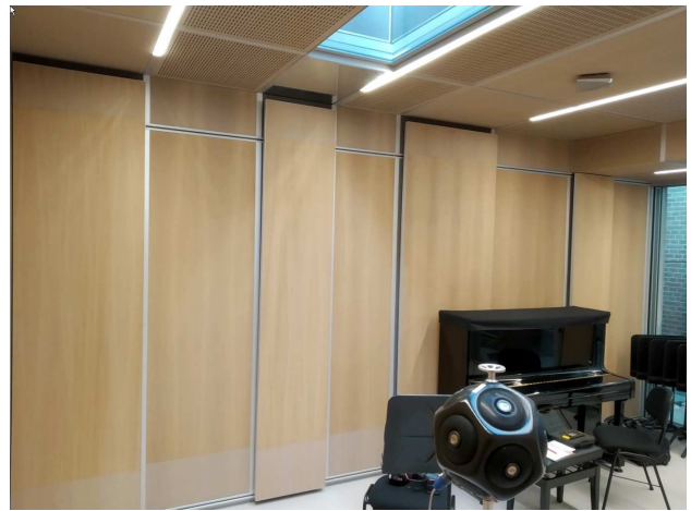
Figure 14. View of wall inside rehearsal room (0.57) for brass players in situation with minimal absorption (sliding reflective panels closed in front of wall absorption).
