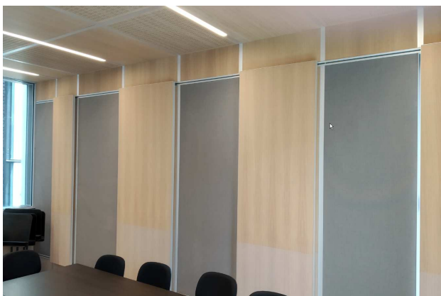
Figure 13. View of wall inside rehearsal room (3.50) in situation with maximum absorption (sliding reflective panels aside of the wall absorption).
