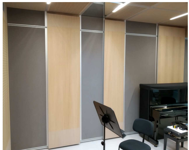
Figure 15. View of wall inside rehearsal room (0.57) for brass players in situation with maximum absorption (sliding reflective panels aside of the wall absorption grey surface).
