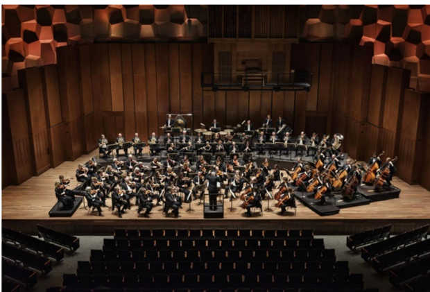
Figure 7. Oosterpoort Groningen: New Stage environment with rotating elements at the rear wall. Also at the side walls of the stage these rotating elements are intended, but not yet implemented.
