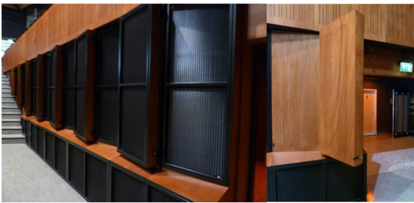
Figure 6. Oosterpoort Groningen: rotating elements at the side walls of the flat floor area, with reflective and absorptive sides.
