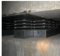
Figure 8 – Elastic bearings in position under dwellings on the pop centre during the construction phase
