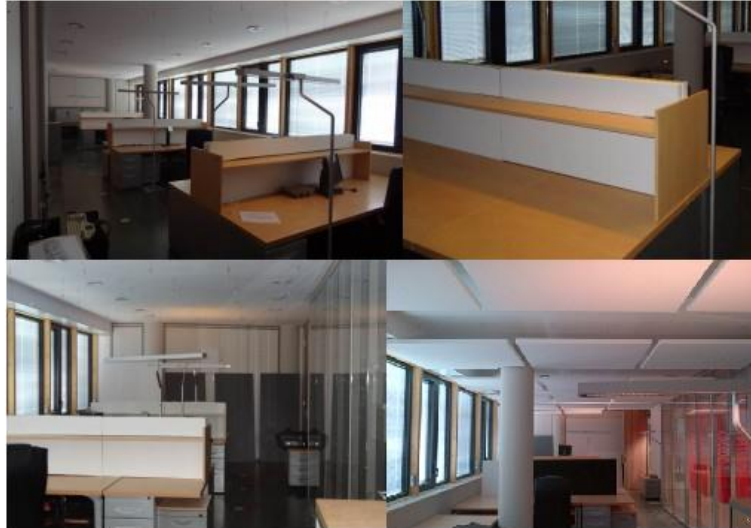
Photograph 2: Top left: Overview of the open-plan office- 0% ceiling coverage ratio; top right: absorptive panels made of high-density glass wool 4cm; bottom left: combination of two absorptive panels against the wall; Bottom right: free hanging units- Ecophon Solo square. Average length 13.7m, average width 4.15m, height under the slab 2.78m. Surface 54m 2 , volume 150m 3 .
