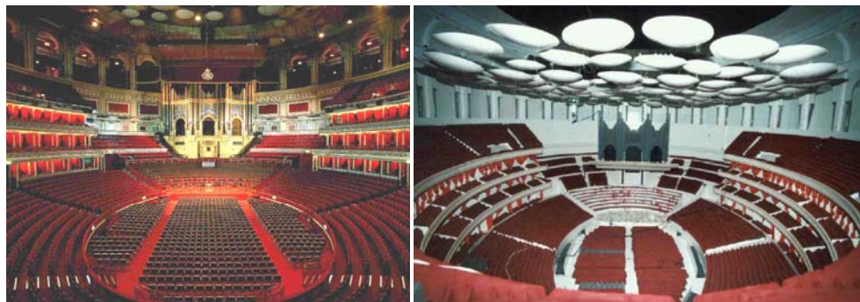
FIGURE 5. Left: interior of the Royal Albert Hall, London; right: Scale model 1:12 with the flying saucers.
