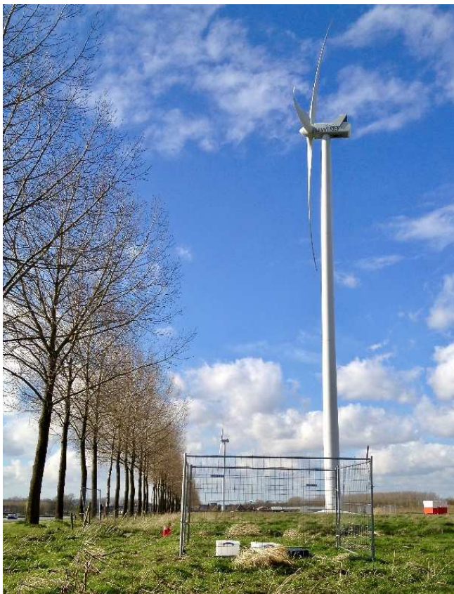
Figure 4: Wind turbine 2 with measurement board in front (inside barrier fence)
