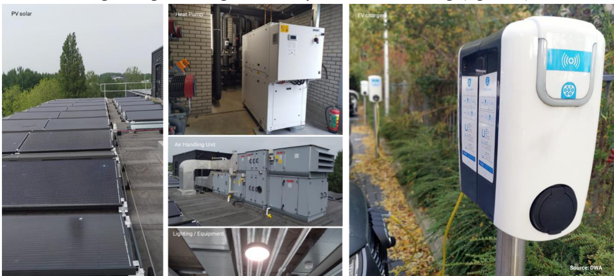
Figure 8.1 Office building DWA.
