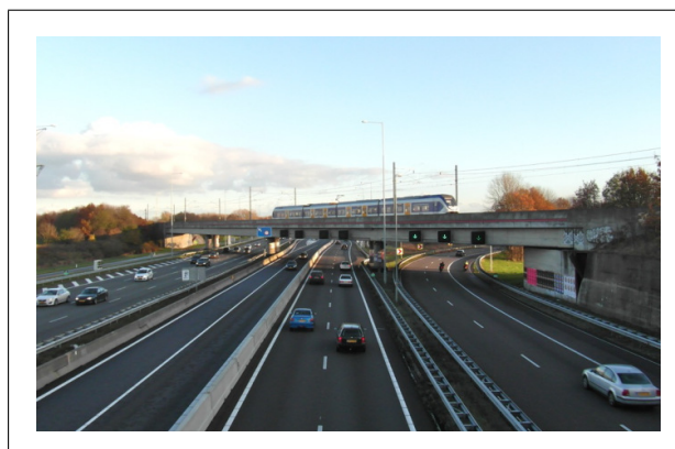
Figure 1. Current railway bridge over the A1 at Muiderberg.
